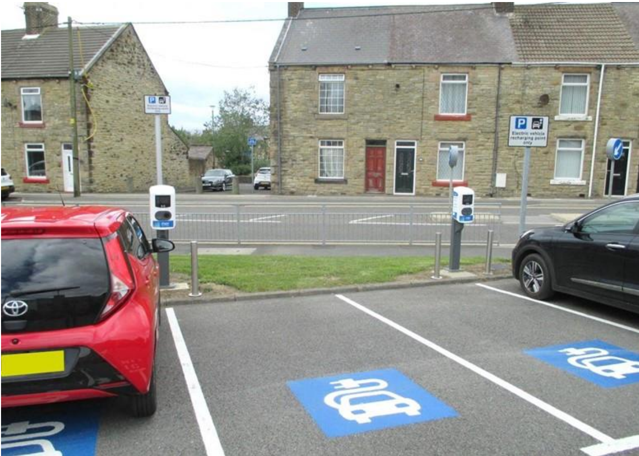
Figure 16: shows chargepoints located in front of four parking bays
