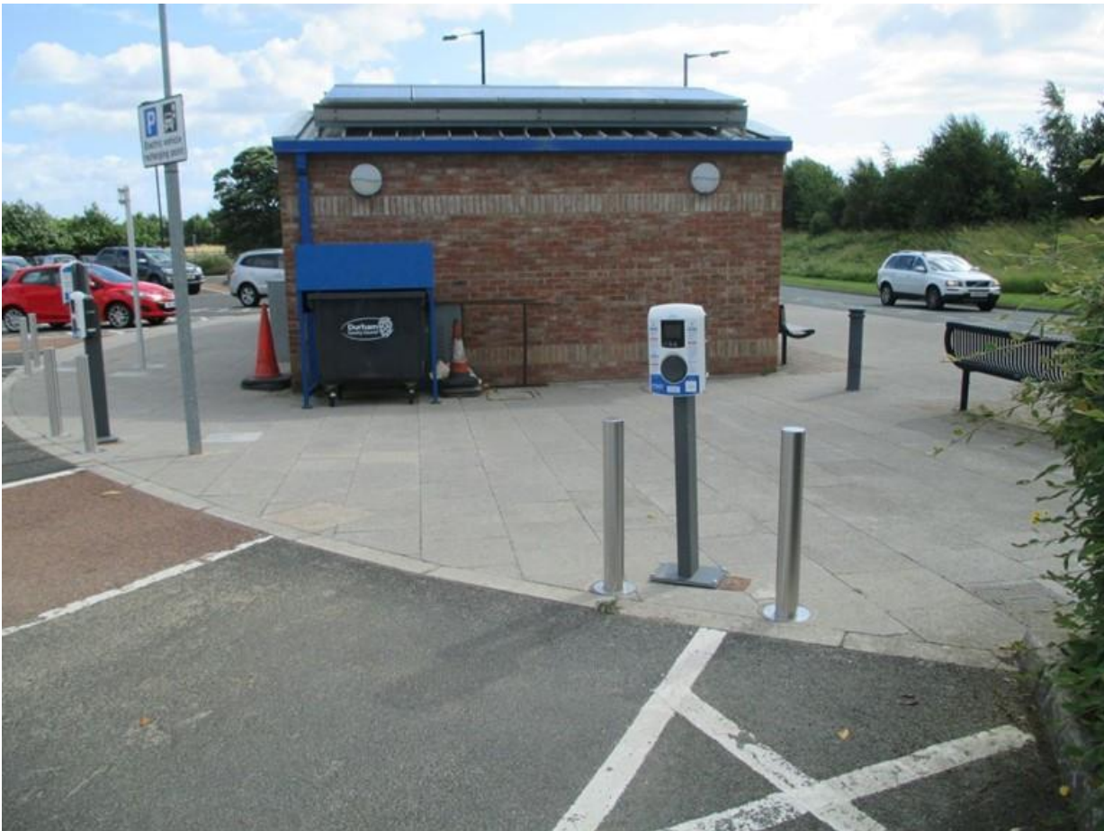
Figure 10: shows a single socket MER Alfen chargepoint
