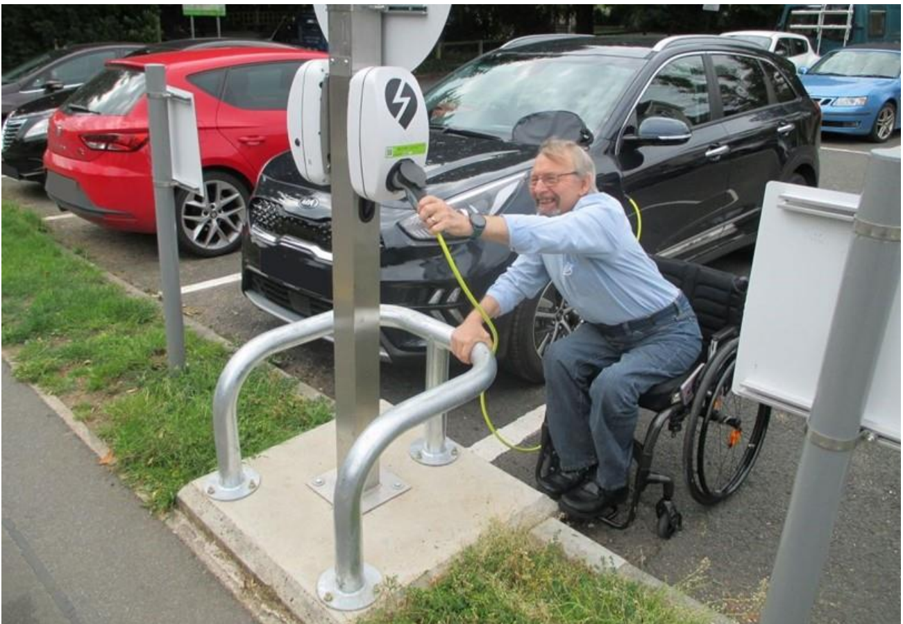
Figure 13: demonstrates difficult access to CMS-EO chargepoint
