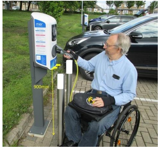
Difference between the existing socket height and this project's proposed inclusive socket height at 900mm above bay level.
