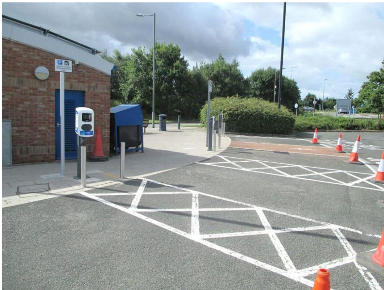
Figure 9: EV charging bays prior to User Trial event
