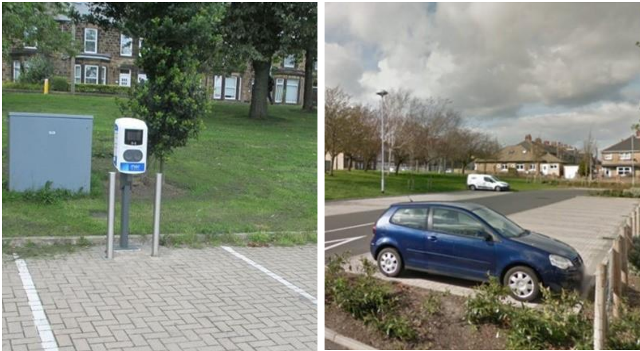
Figure 11: MER-Alfen twin socket chargepoint in vehicle bay & Pre-installation
