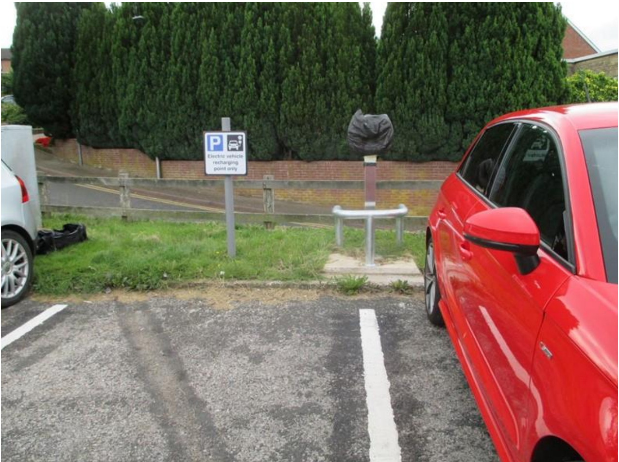
Figure 15: shows the chargepoint location in front of two parking bays
