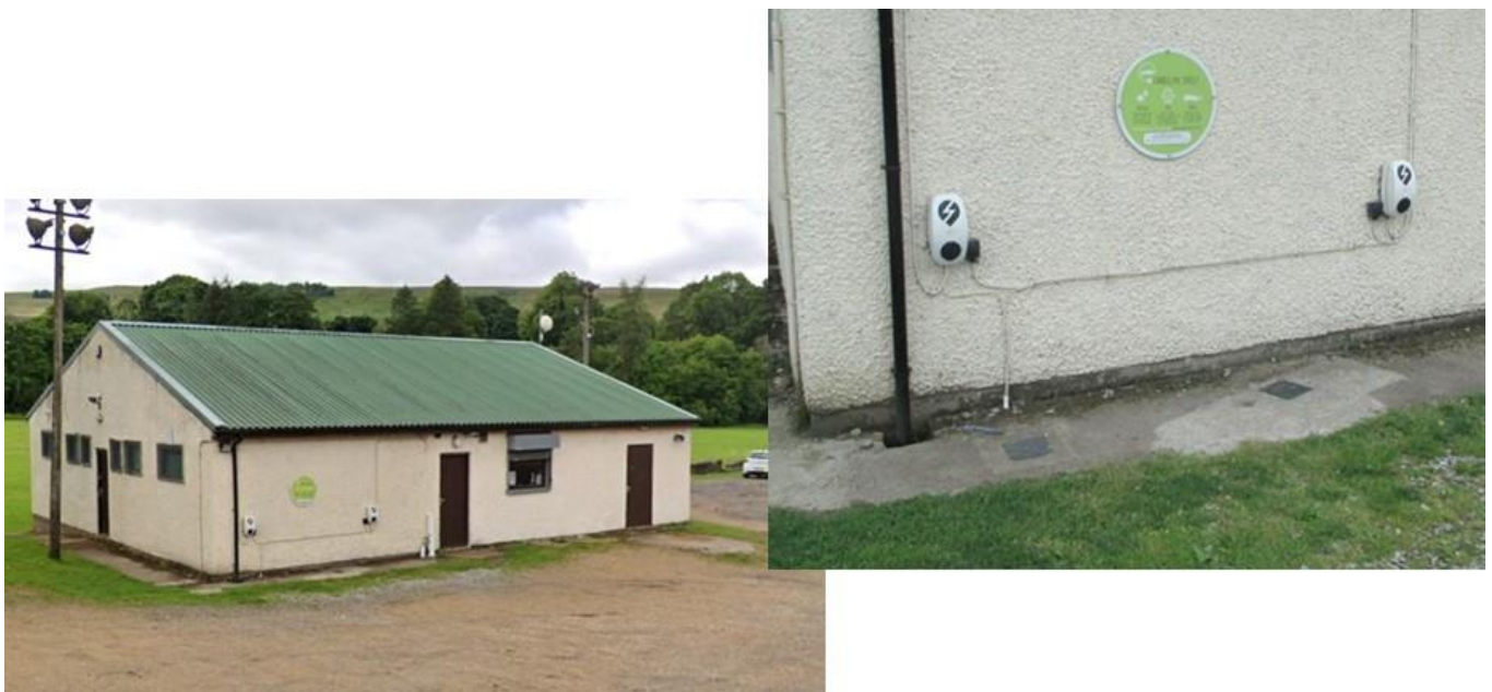
Figure 18: shows the two wall-mounted Charge My Street chargepoints
