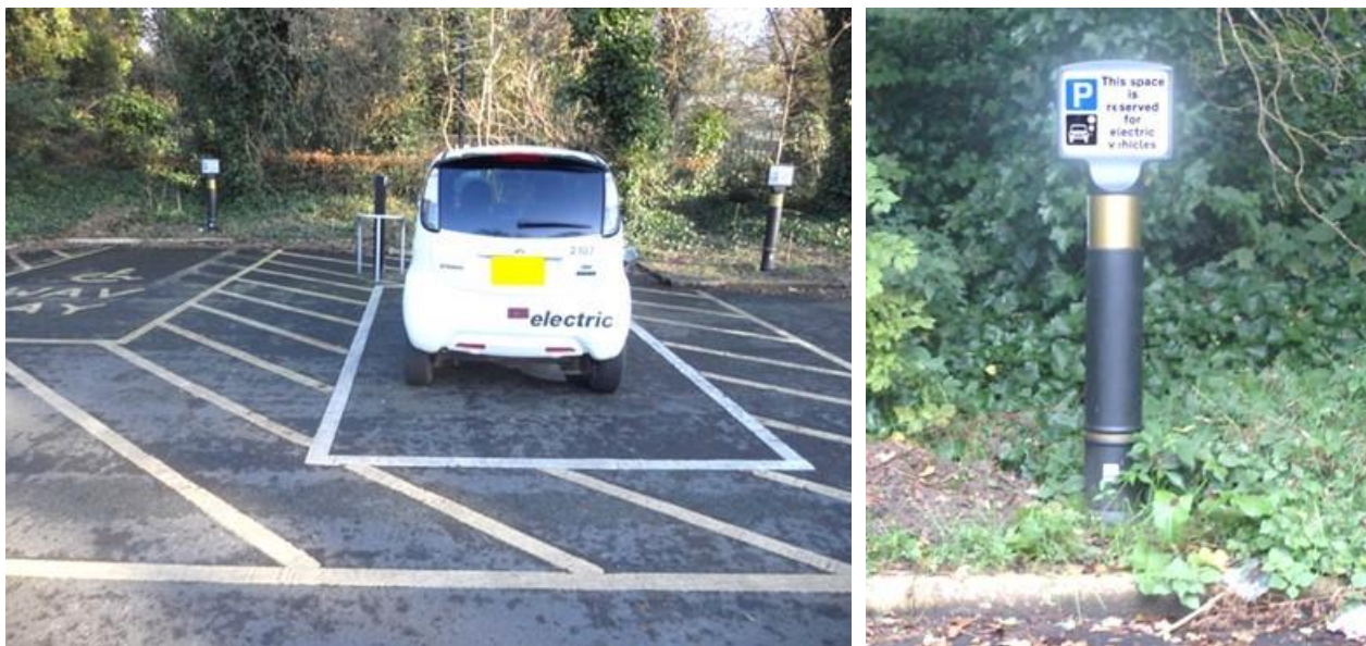
Figure 5: Level access EV Bay & Signage
